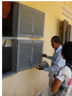
Window hinges to change from vertical opening (left) to side opening (right)
