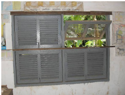
Window hinges to change from vertical opening (left) to side opening (right)
